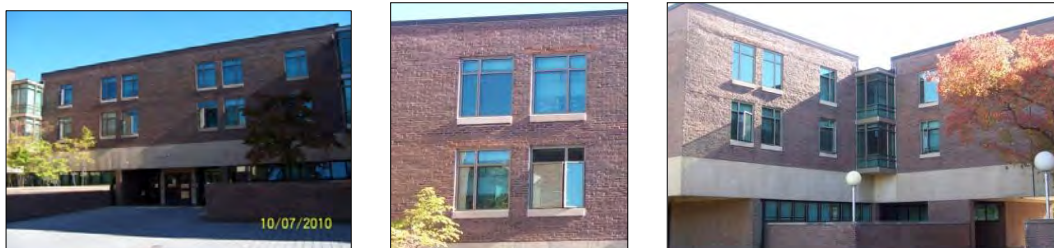
Exterior views of window replacement
