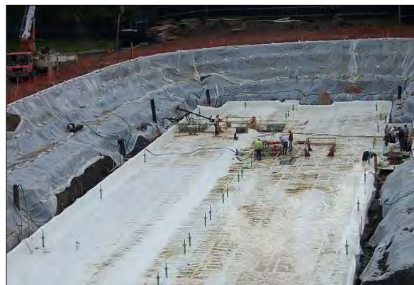
Installation of waterproofing
