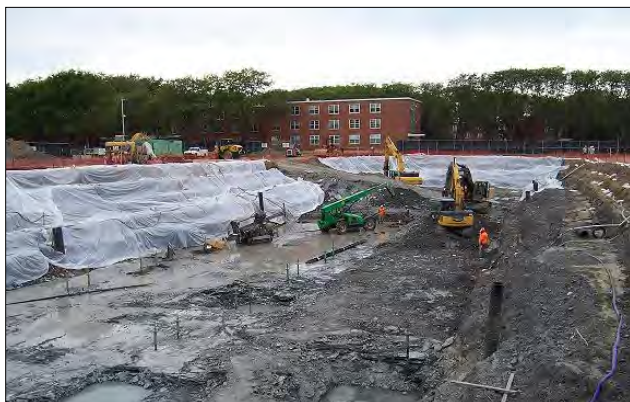
Excavation of basement and foundations
