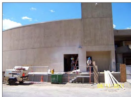
Construction of loading dock/service entry
