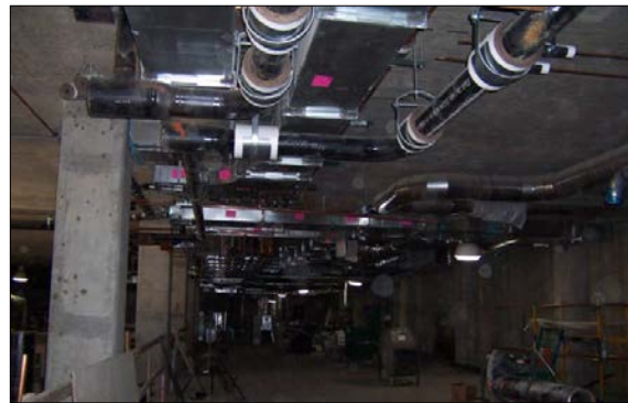
Mechanical and Plumbing Work In Basement
