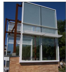
Exterior Wall Mock-Up
