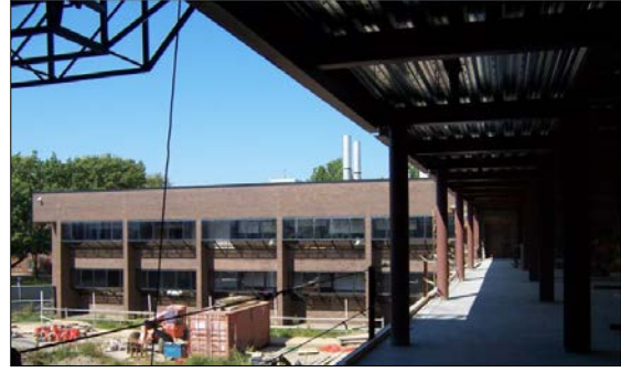
Second Floor Connection to Houghton Hall
